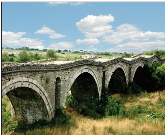
Bridge of Terziu
